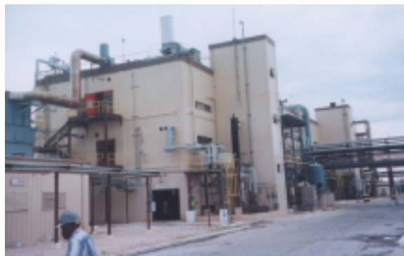
Plant 1-Multipurpose Facility
